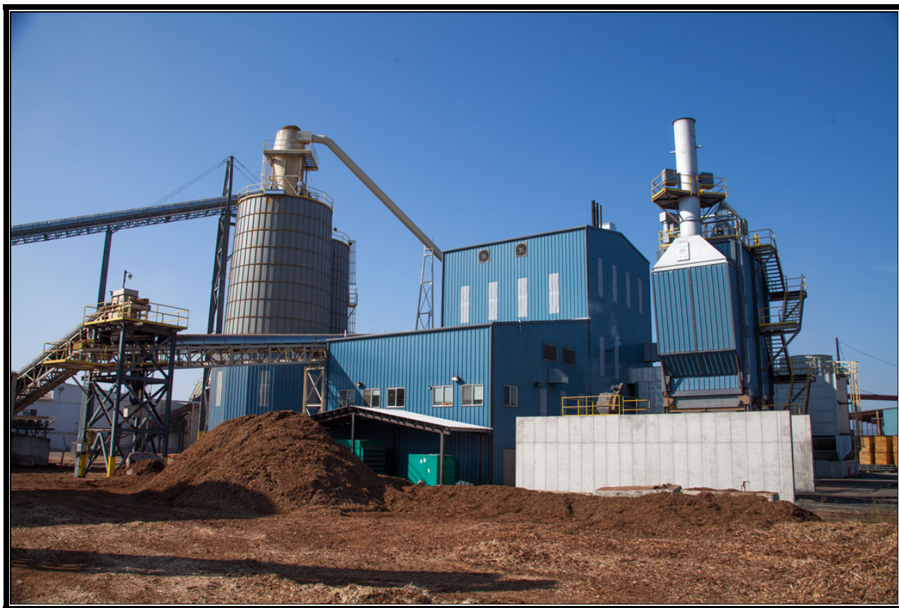
Figure 4.1A – 3 MW Boiler/Steam Turbine Cogeneration Power Plant
