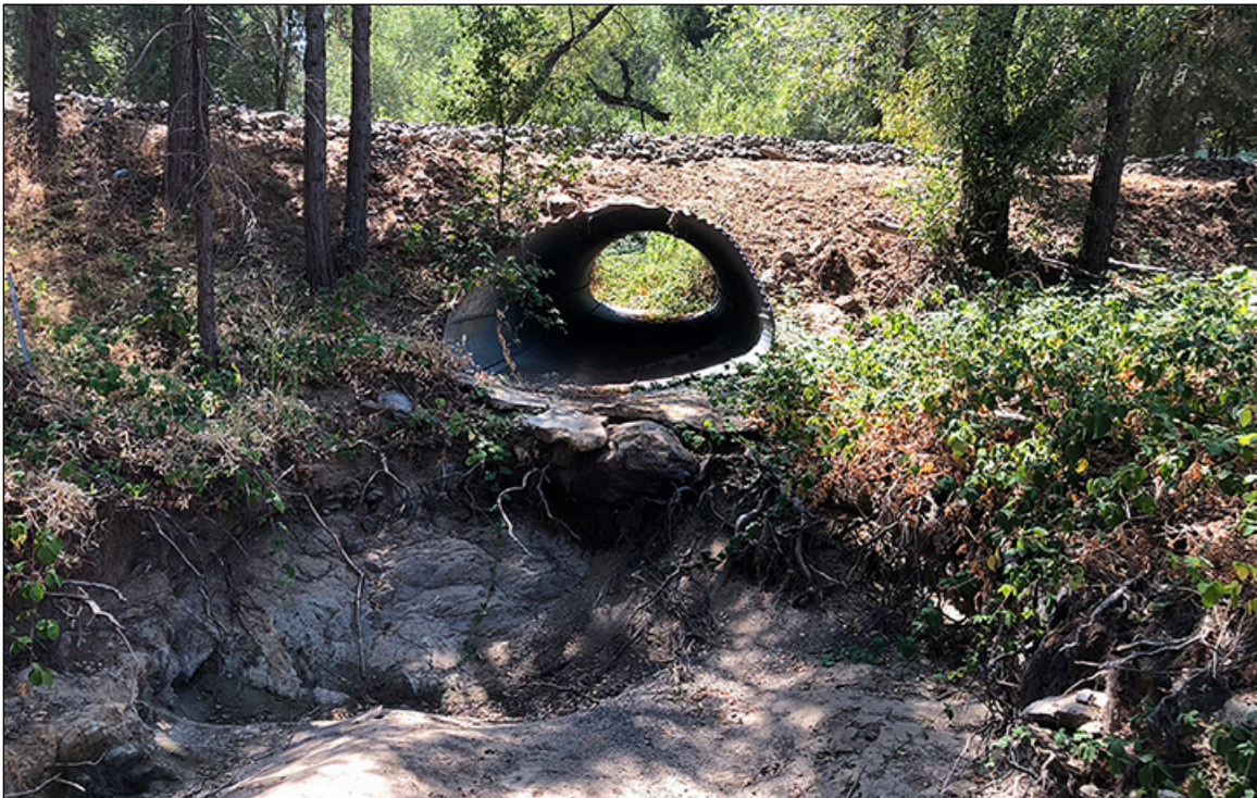
Photo 12. Groveland west parcel - Culvert under the Groveland Community Service District access road showing scouring pool.
