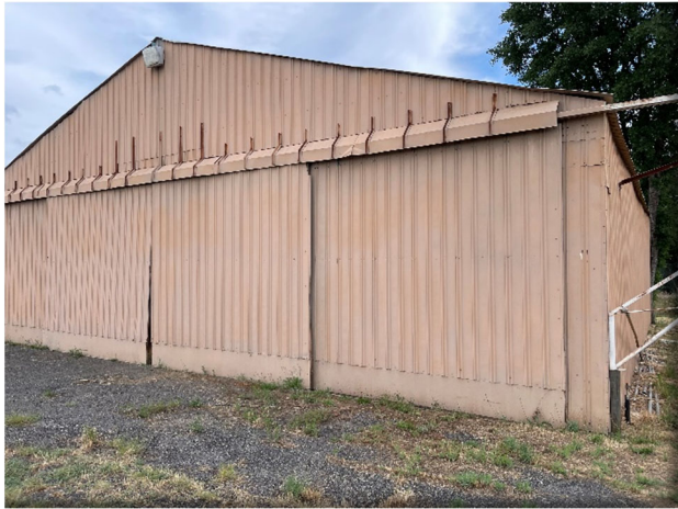
Executive Hangar Fickel Box Hangar
