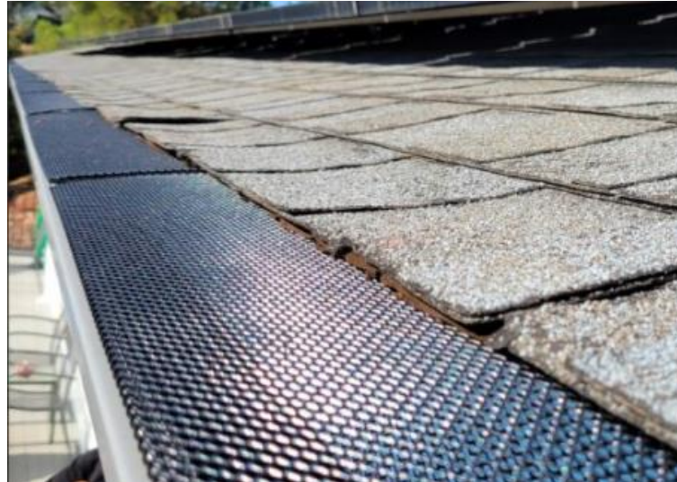
Noncombustible Gutter and Cover
