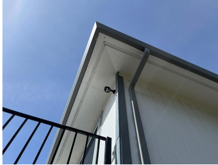
Enclosed Eaves with WUI Soffit Venting
