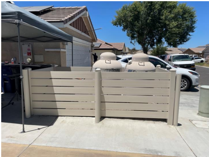
Metal Propane Enclosure
